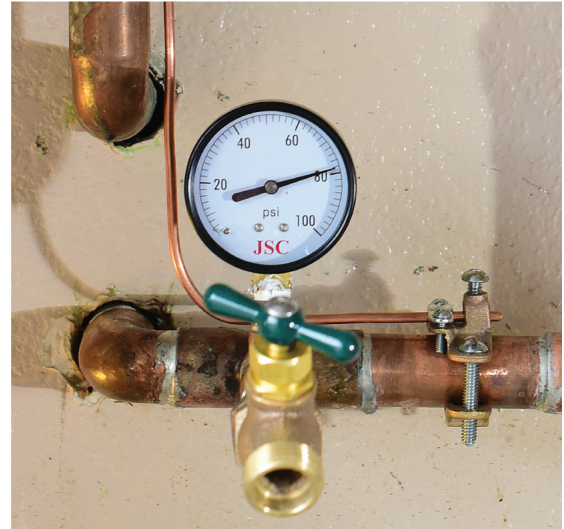
Figure 8 - Copper wire clamped to incoming water main
